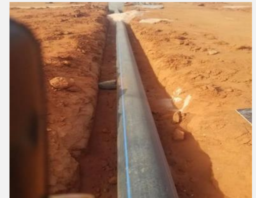
HDPE water pipe layed in prepared trench
