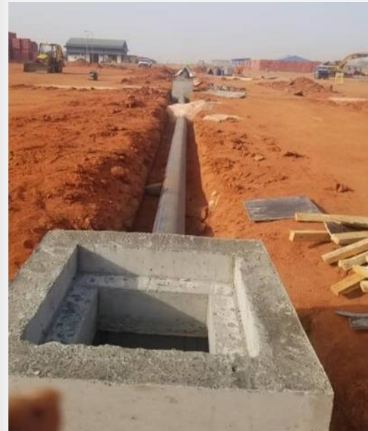
HDPE pipes layed and connected to chamber
