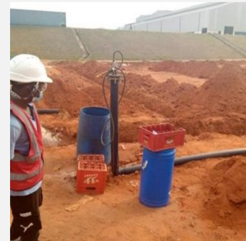
Pressure testing of welded HDPE pipes
