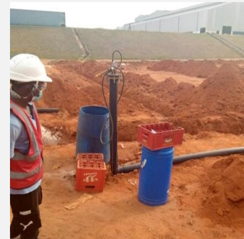
Pressure testing of welded HDPE pipes
