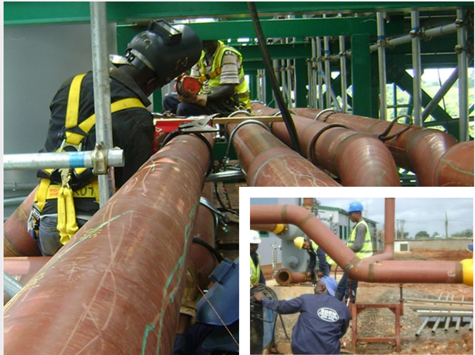
Prefabrication and installation of piping works for W18V50DF engine.
