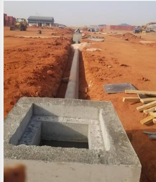
HDPE pipes layed and connected to chamber
