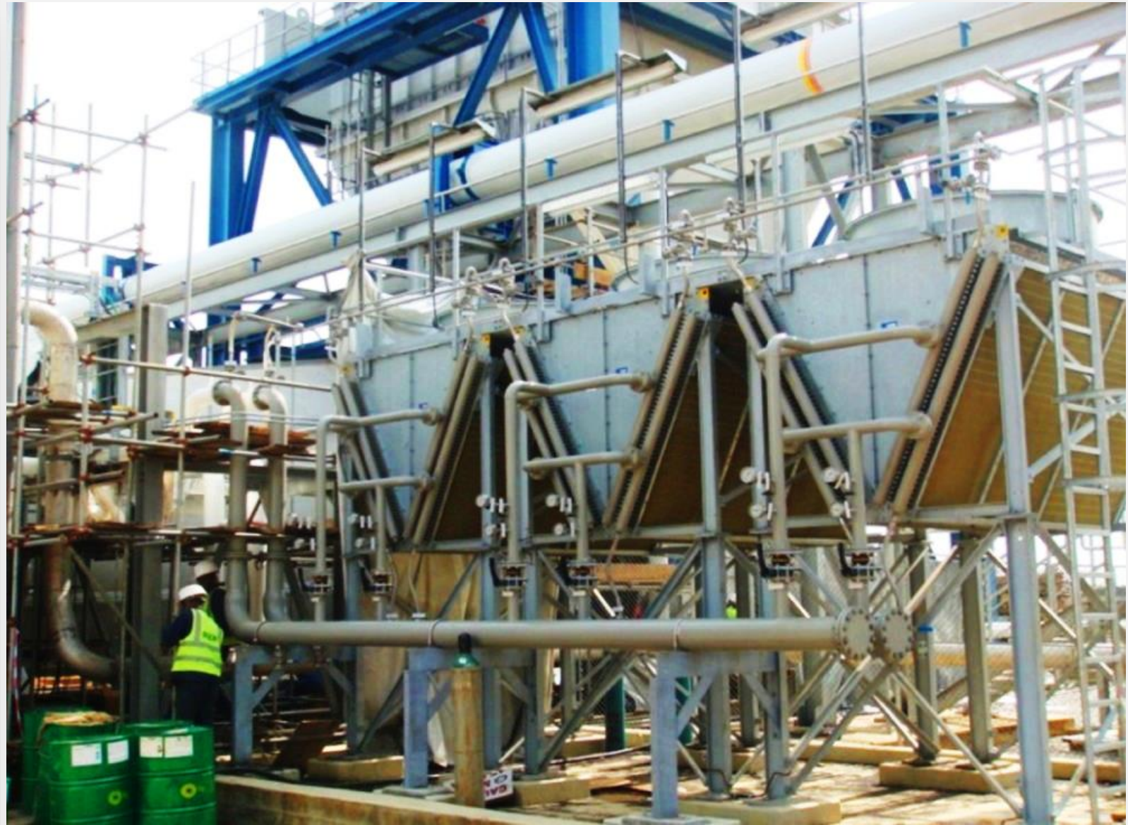
BOP installation (cooling water system).
