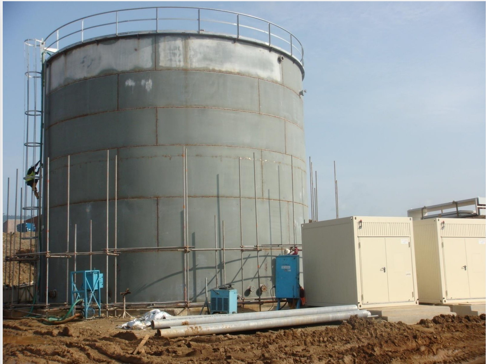
Storage tank: raw water tank fabrication in progress
