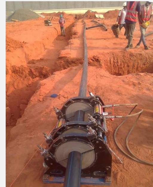
Butt fusion joint welding of HDPE water pipes
