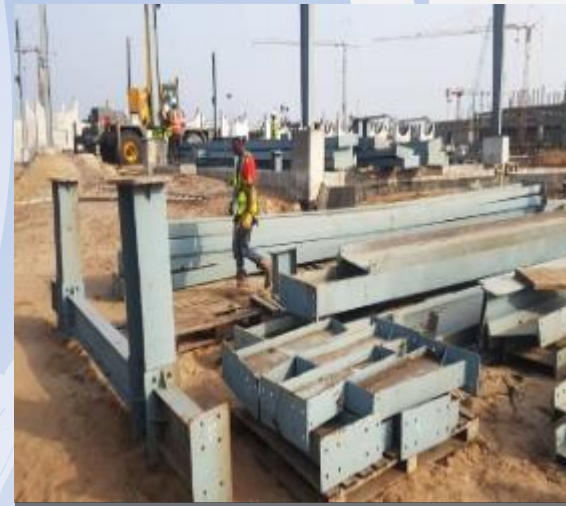
Associated steel structures (supply, fabrication & erection)
