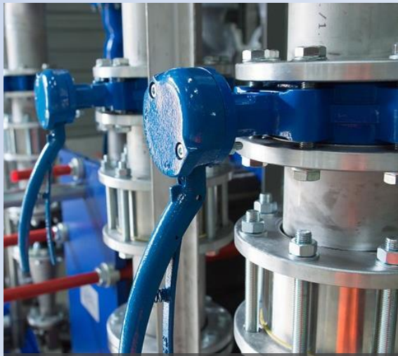
Valves (supply & erection)
