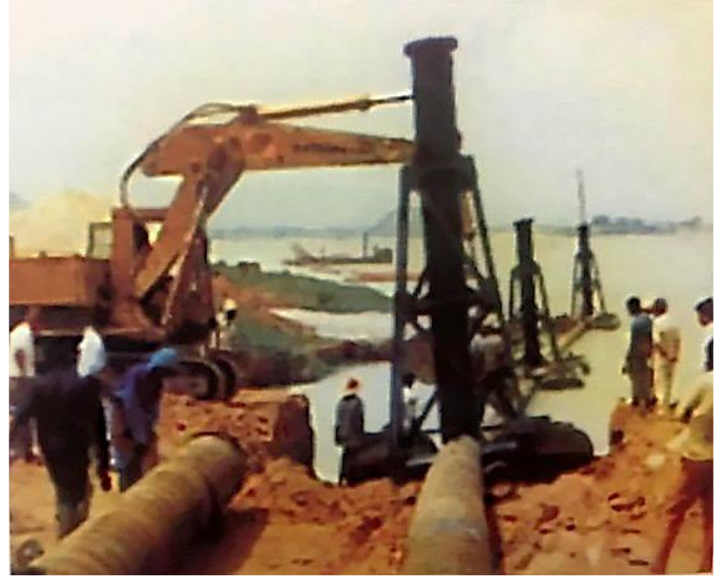
Project: Water intake, main distribution lines (18Km) and water storage tank
