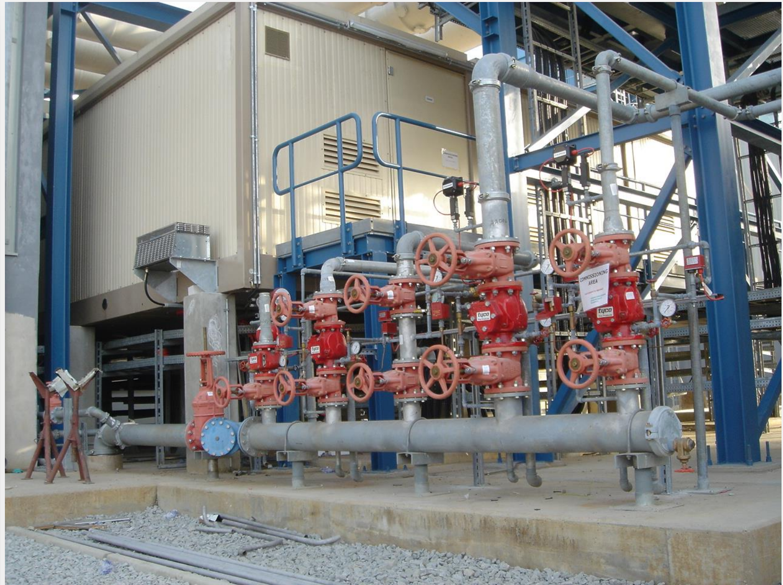
Water piping bypass network
