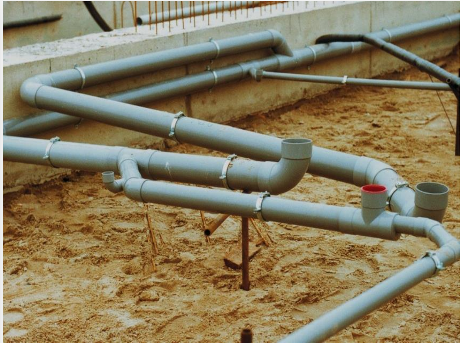
Light weight PVC-U system Installation
