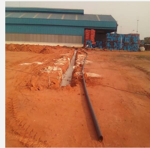
Prepared excavated trench surface ready to receive HDPE water pipe
