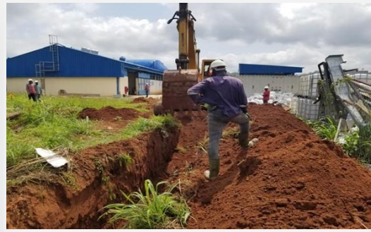
Excavation of trench for HDPE water pipeline using sdem excavator
