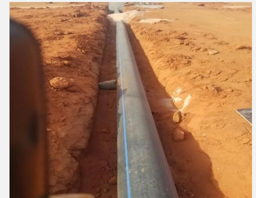
HDPE water pipe layed in prepared trench
