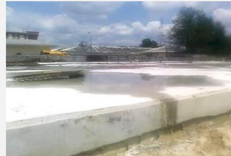
Concreting of Ground floor slab completed
