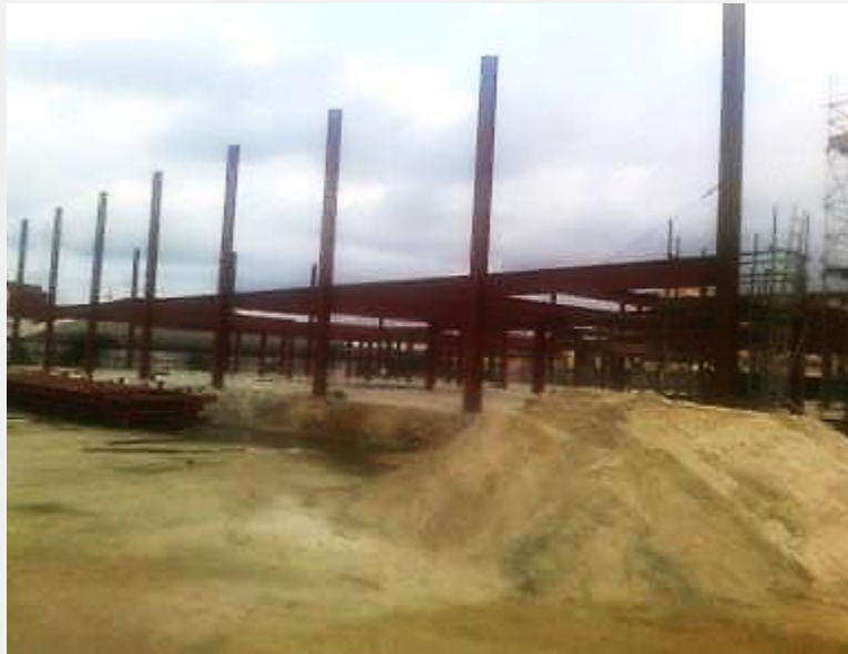
Erection of steel structure commence
