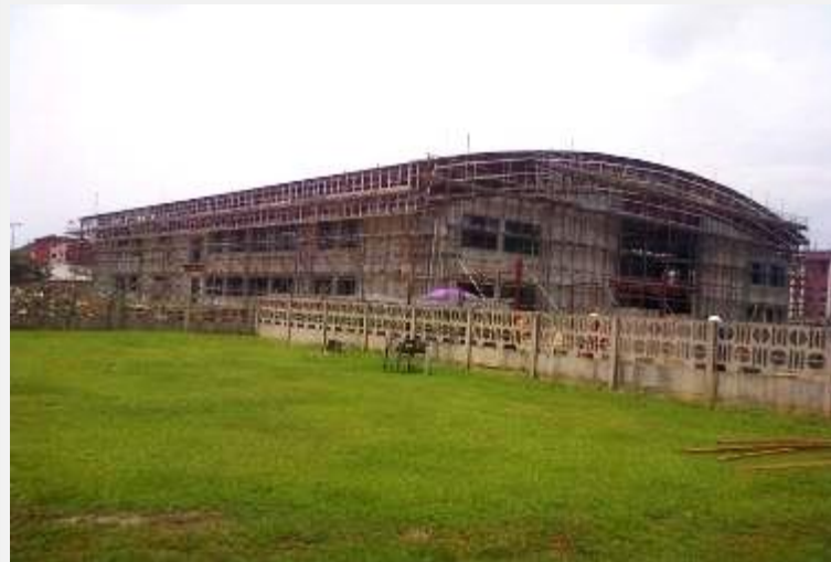
External and Internal block work completed and roofing sheet installed
