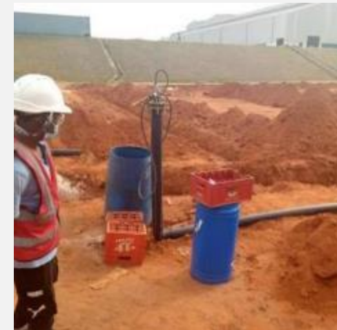
Pressure testing of welded HDPE pipes
