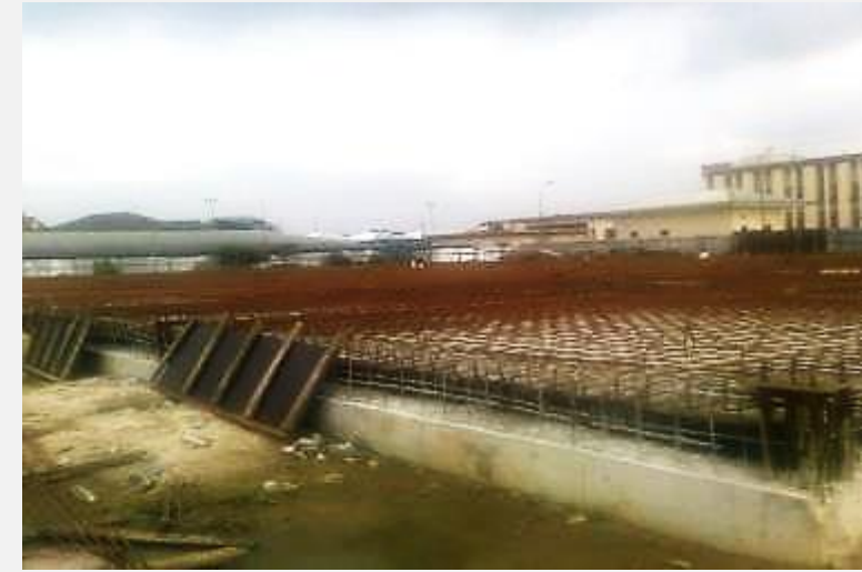
Ground slab Re bar, formwork and anchor bolts installed
