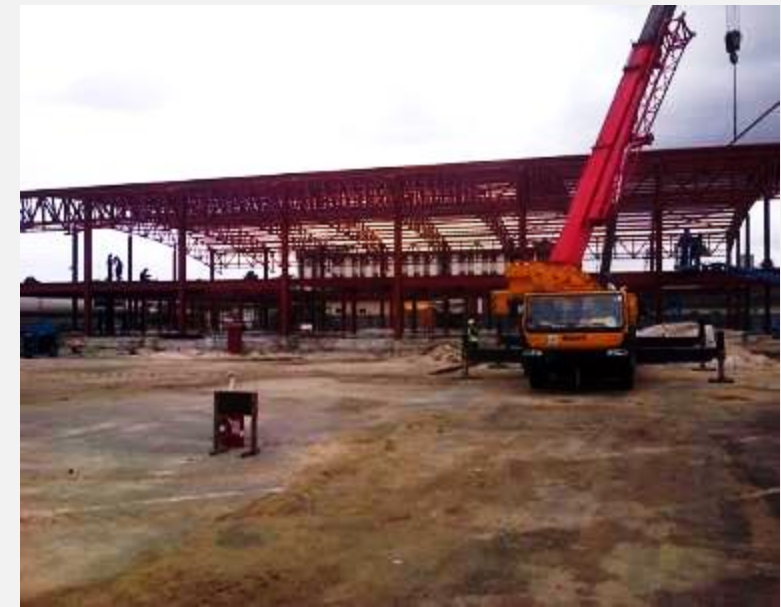
Erection of steel structures continues
