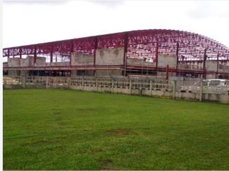
External block work on going
