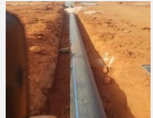
HDPE water pipe layed in prepared trench
