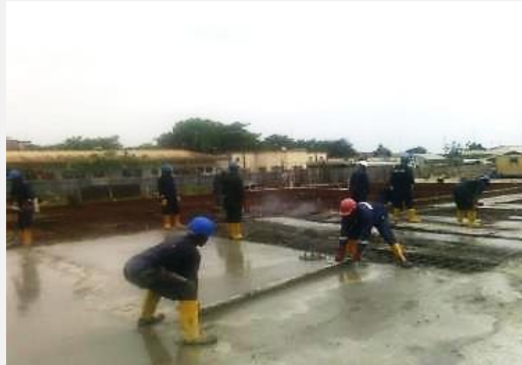
Concreting of ground slab In progress
