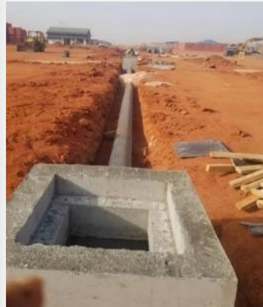
HDPE pipes layed and connected to chamber
