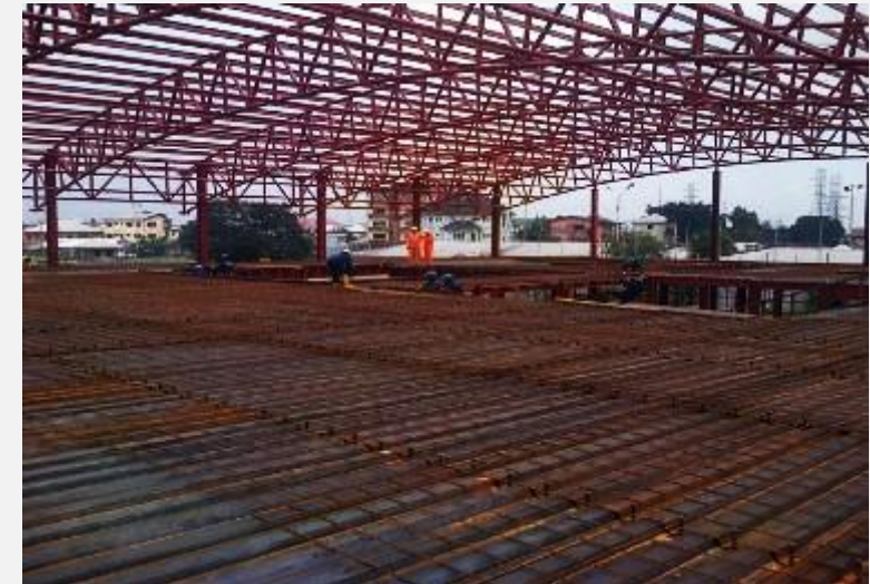
Installation of studs and metaldeck plate to receive concrete completed
