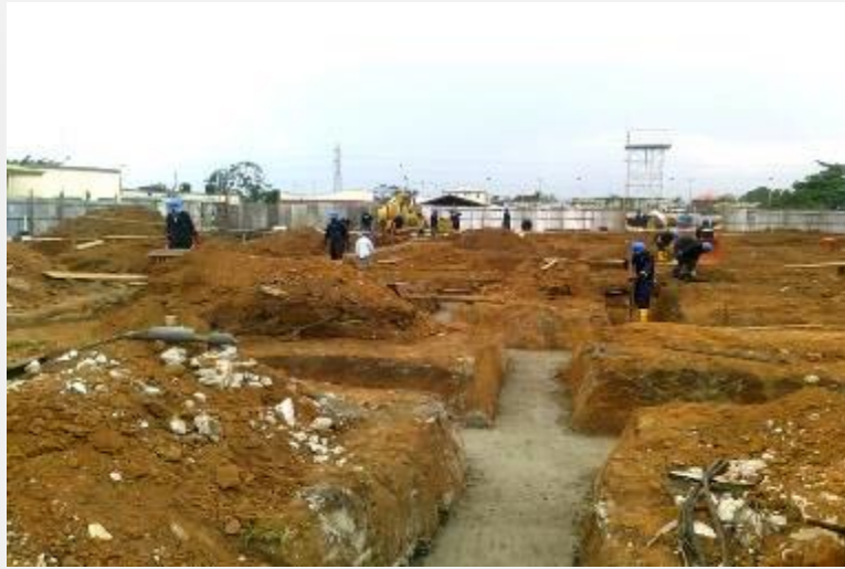
Foundation strip excavation & blind completed
