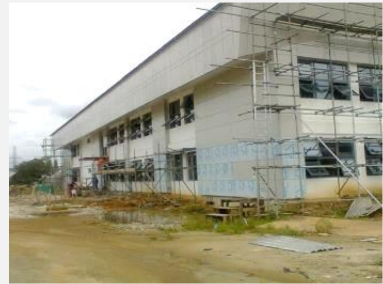
Cladding and painting of external wall
