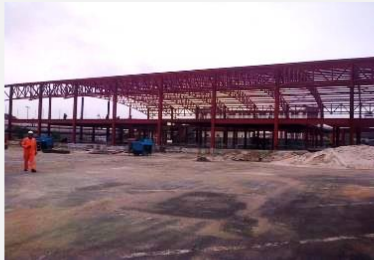
Erection of steel structures completed
