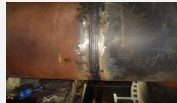
Welding of 21" Diameter High Pressure Steam Pipe (1.1/4" thick).
