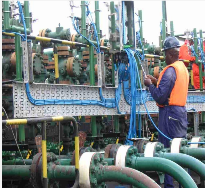
Instrument Cable laying at an offshore flow station
