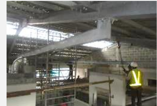
Warehouse MEP steel works in progress.
