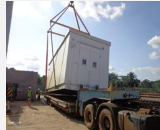
Transportation, Lifting & Installation of Control room for the Gas Plant.
