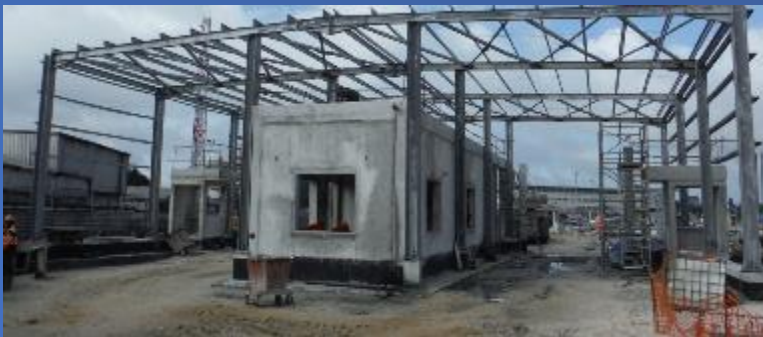
Erection of hot dip galvanized steel structure.
