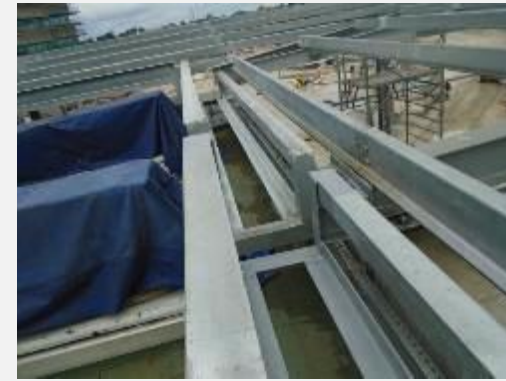
Installed gutter rails & purlins at the top basement.
