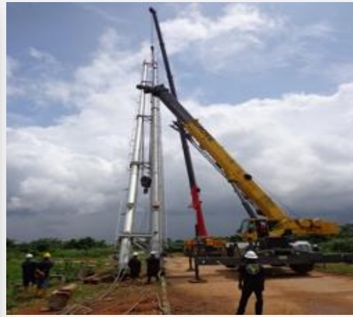
Tandem Lifting & Positioning of Flare Stack c/w guy wires and accessories.
