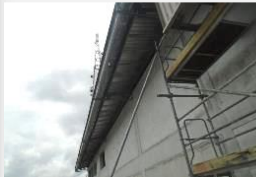
Installed Drain at view from the south.
