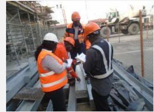
Material Inspection after delivery to site.
