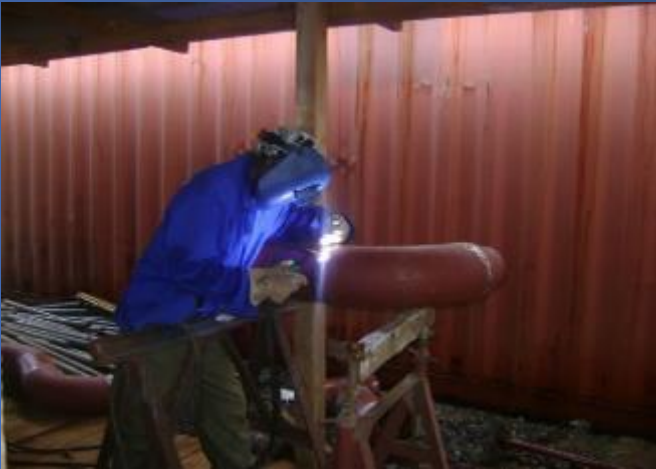
Fabrication & TIG Welding of gas pipe spools.
