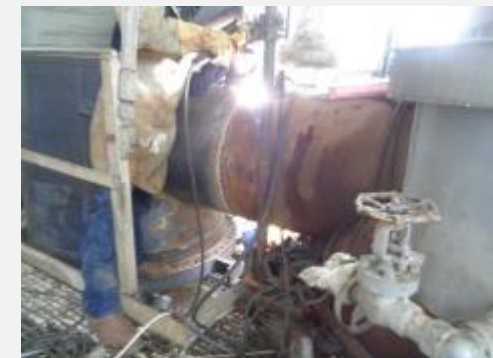
Welding of 21" Diameter High Pressure Steam Pipe (1.1/4" thick).
