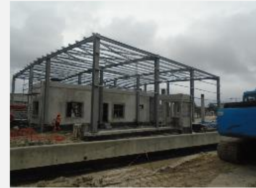
Erected transit gate house awaiting roofing.
