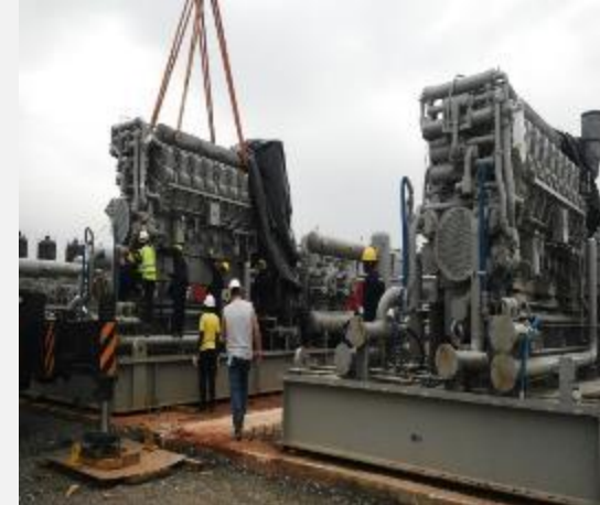
Lifting & Installation of 6Nos Cartapiller Gas Re-compression Engines and Compressor Skids on respective Foundations at gas Plant.
