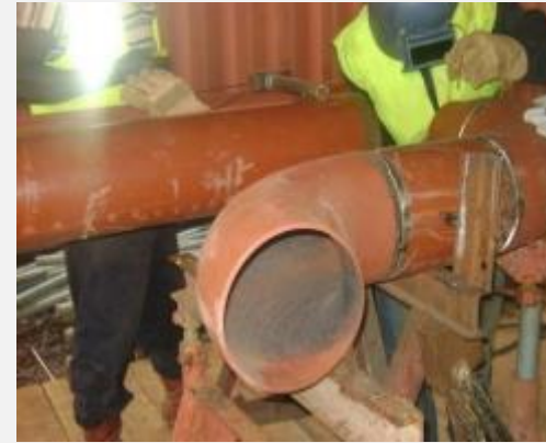
Pre-fabrication of fuel gas header spools.
