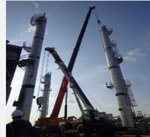
Lifting & Installation of Debutanizer, Depropanizer & Deethanizer Towers c/w Steel Platforms, Access ladders, Interconnected piping systems & Reflux Condensers.
