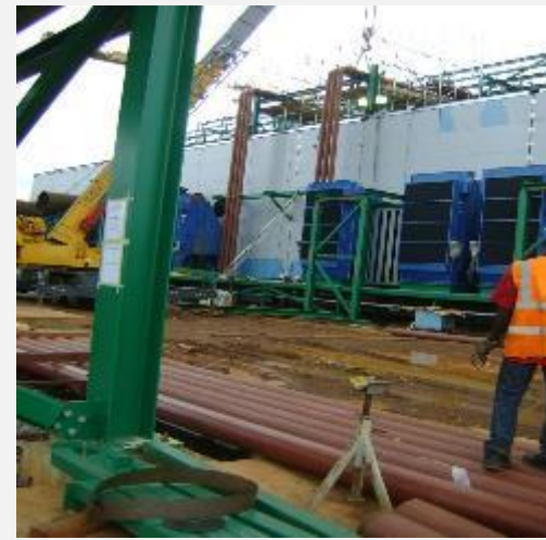
Bop/Piping Installation For W18V50DF (100MW) Gas Engine Power Plant,
