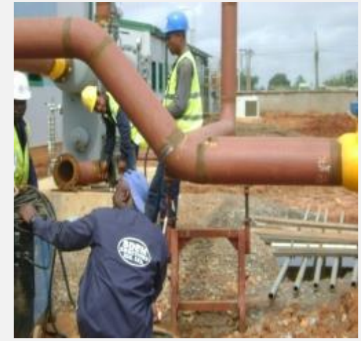
Bop/Piping Installation For W18V50DF (100MW) Gas Engine Power Plant,
