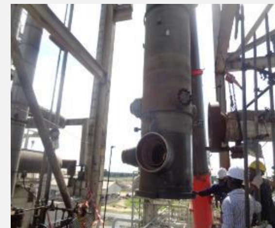
Positioning of the 101C Boiler before welding of auxiliary piping systems and connection of appurtenances.
