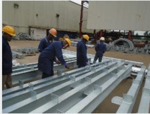
Process Inspection and documentation during galvanization.
