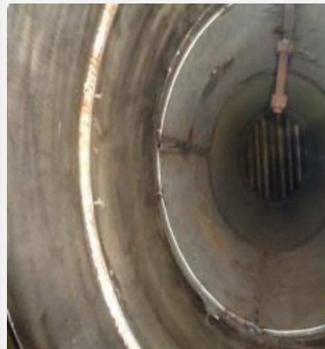
Internal fracture repairs of High-Pressure Boiler Casing.
