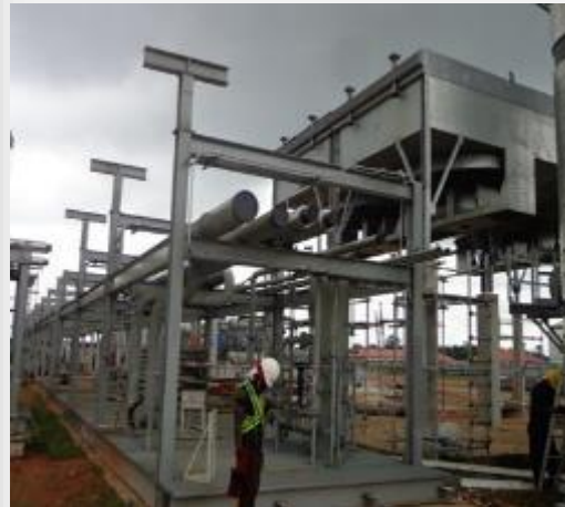
Lifting & Installation of pre-fabricated Pipe supports, Walkways, Pipe spools, Gas Valves and Instruments.
