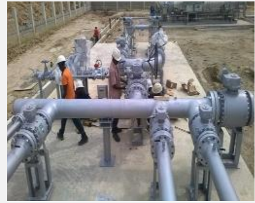
Piping system installation for Gas Metering Station.
