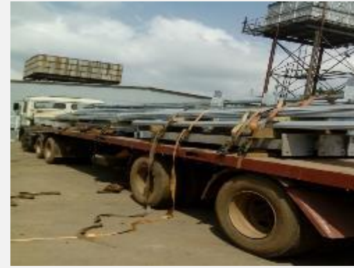
Materials transportation and stacking.
