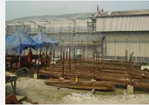
Newly extended warehouse building with roofing commenced.
