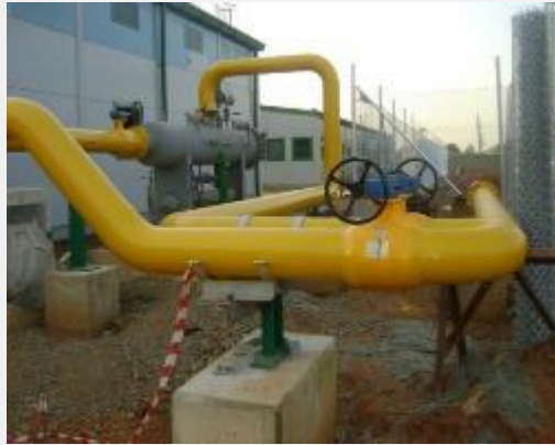
Fuel gas header hook-up.
