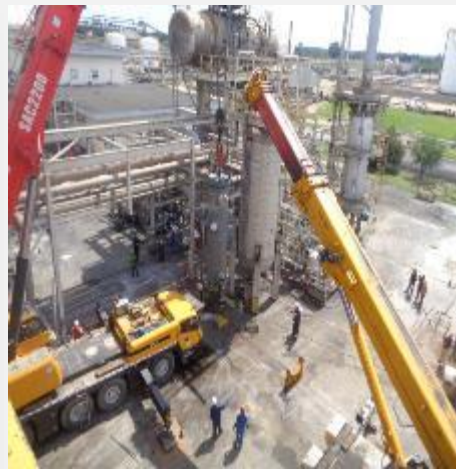
Tandem Lifting of new 101C Boiler for Notore Ammonia Plant.
